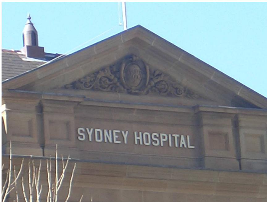
Photo 4. PEDIMENT TO GABLE OF SYDNEY HOSPITAL, MACQUARIE STREET
