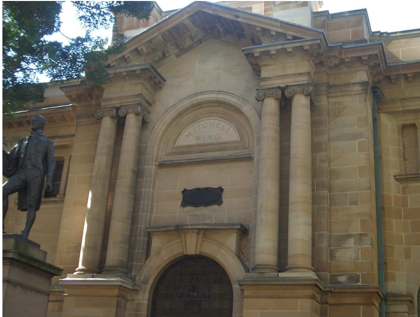
Photo 5. IONIC COLUMNS TO ART GALLERY, MACQUARIE STREET
