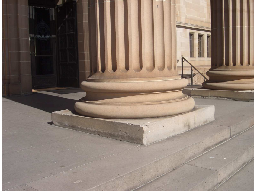
Photo 9. IONIC BASE TO ART GALLERY, MACQUARIE STREET
